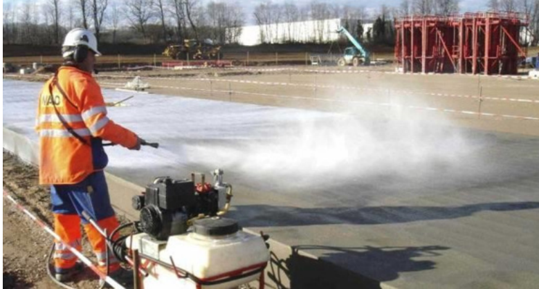
Fig. 7: Membrane Curing
